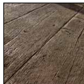
Gilpin's Falls Bridge Plank
